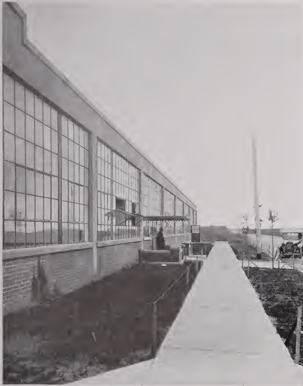
WORKS ENTRANCE TO MAIN FACTORY
